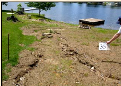
Examples of Identified Erosion Problems
